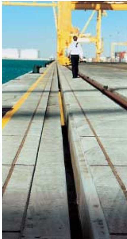
Jebel Ali Port - Dubai. The pre-existing slot used for the Panzerbelt installation.
