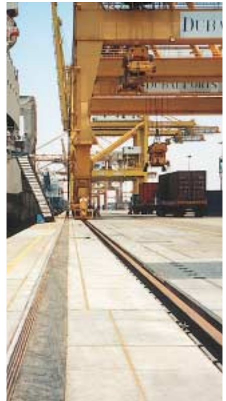
Jebel Ali Port - Dubai. The finished retrofit installation 1500 m long.
